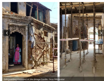
Safeguarding measures at site (Image Credits: Zeus Pithavala)
